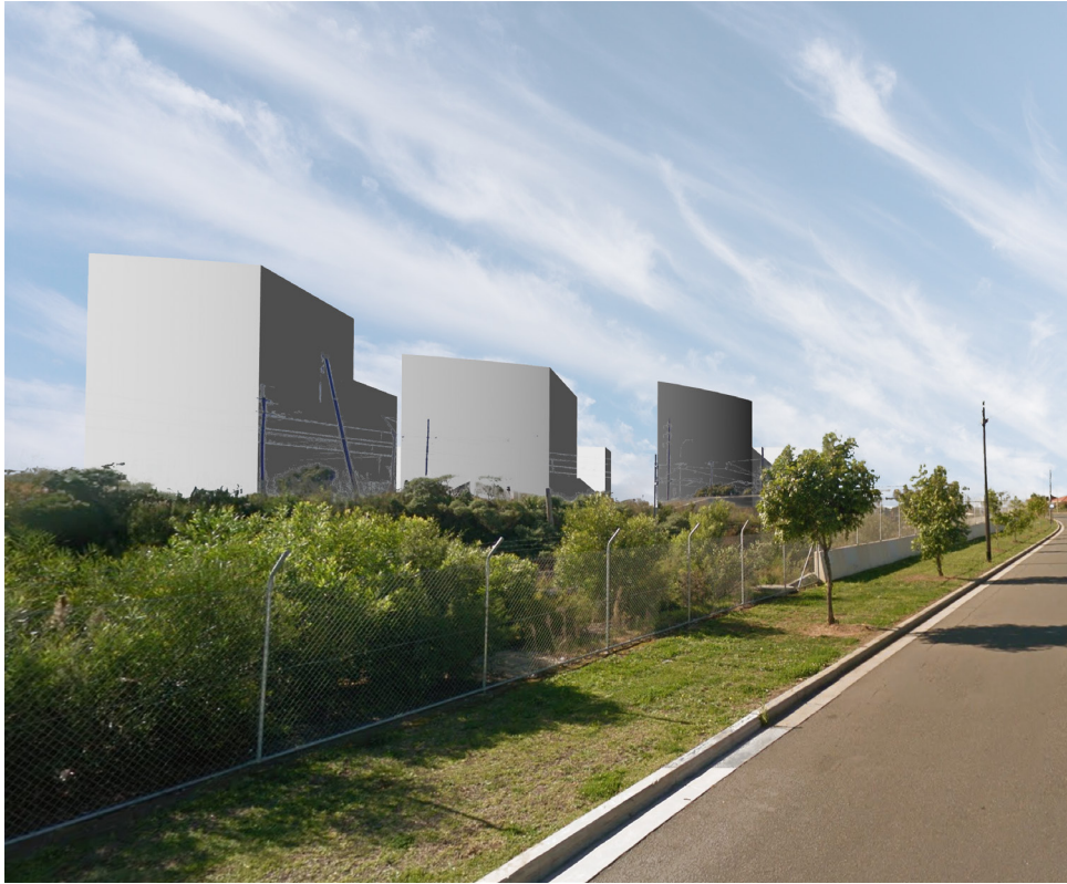
Ⓓ Fig. 1 View from Wellington Rd
