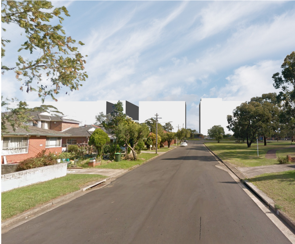
© Fig. 1 View from Morris St
